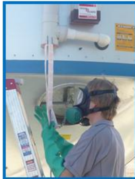
Insert Bag Chain into Chamber
